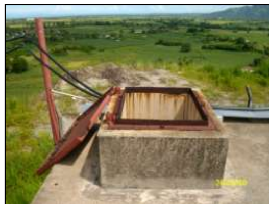
Rusted open inspection chambers
