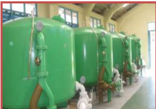
Buabua Treatment Plant- Pressure sand Filter
